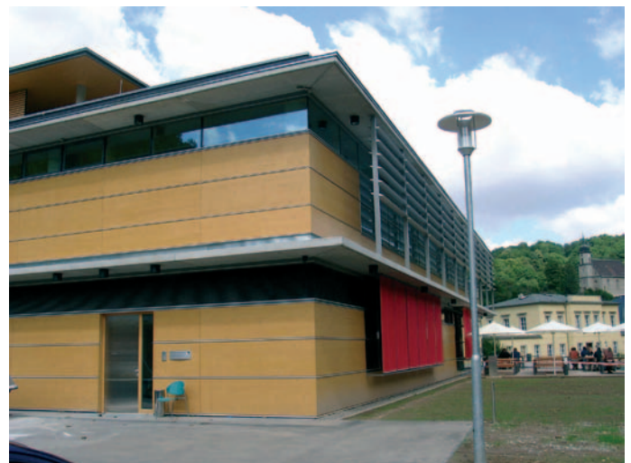
October 2005: The centrally situated new building of the Tharandter Campus houses the Branch Library of Forestry Sciences as well as the refectory.
